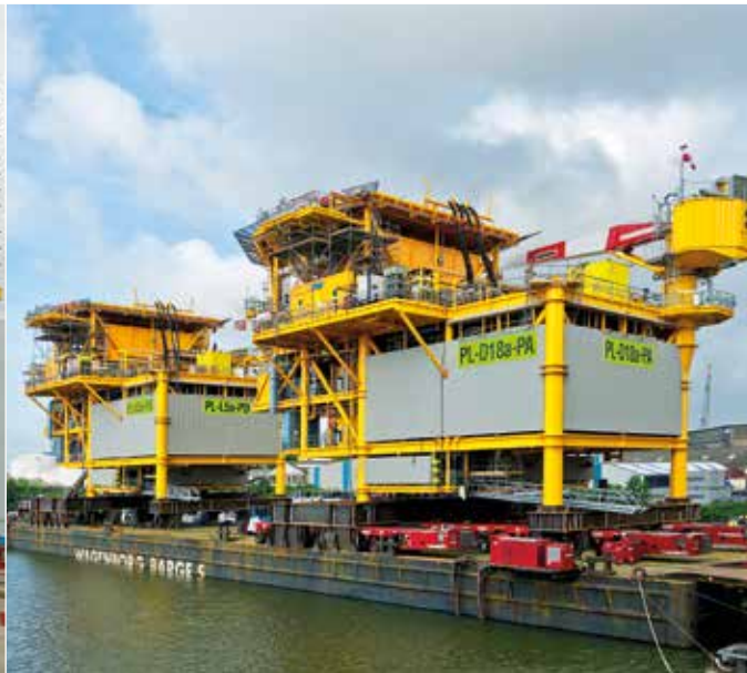
Two gas platforms delivered within one year
