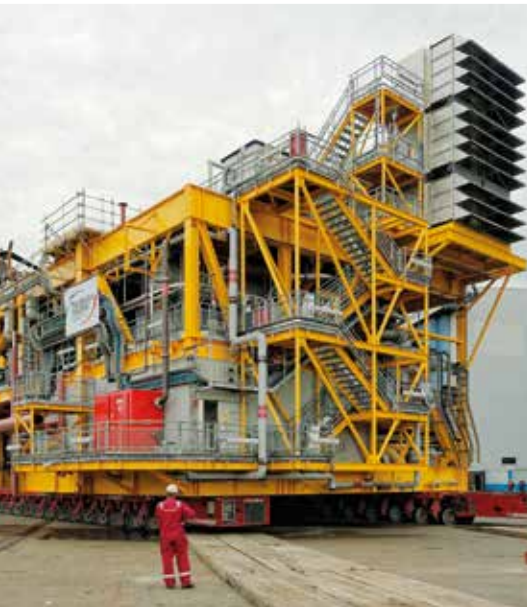
Compression module 1,600 tonnes
