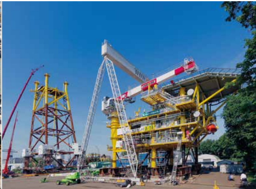
EPCI gas platform
