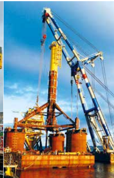
Re-usable platform with suction piles
