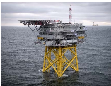
Borkum Riffgrund – installed
