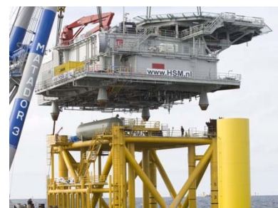
Horns Rev B - installation of topside
