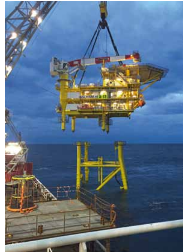
Installation of A18 satellite platform for Petrogas E&P Netherlands.
