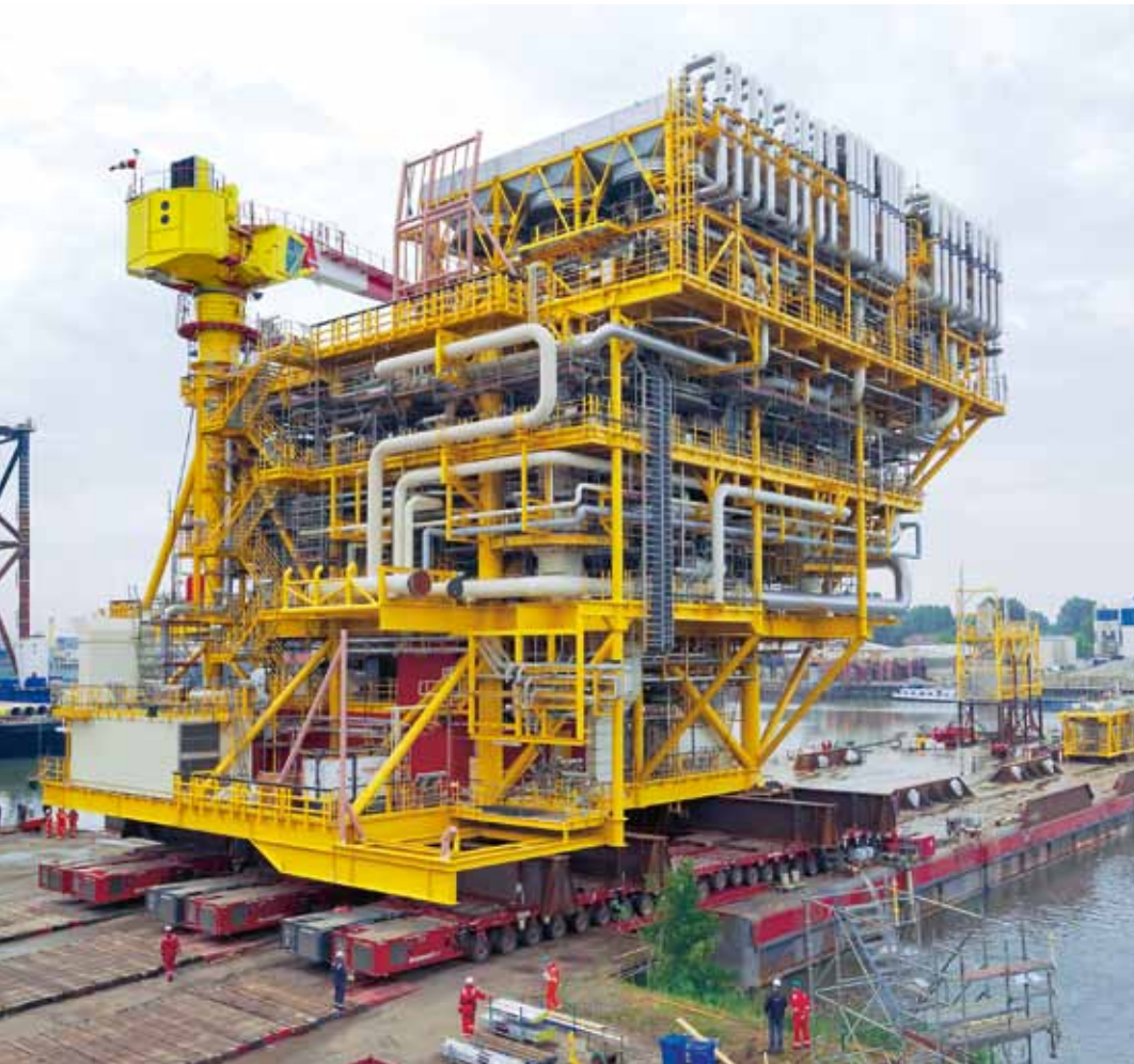
Load-out of Shell Leman Uptime compression platform at HSM yard.
