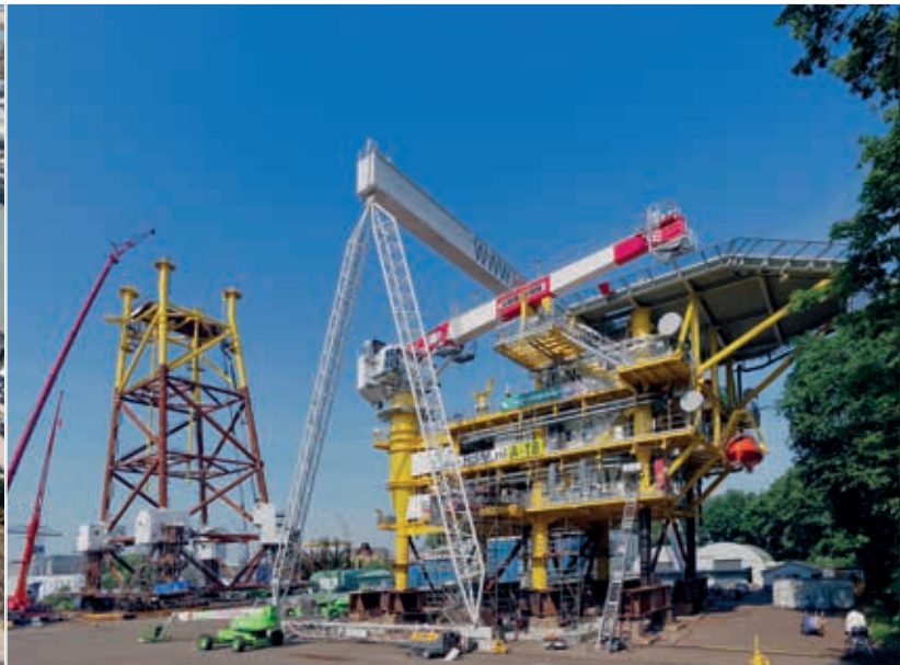
EPCI gas platform
