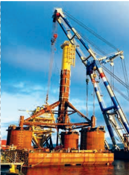
Re-usable platform with suction piles
