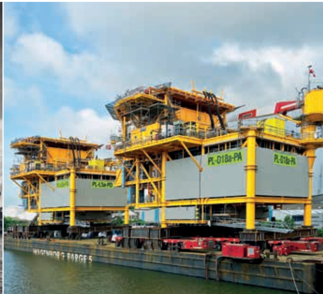
Two gas platforms delivered within one year
