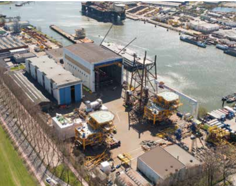
HSM Offshore facilities in Rotterdam harbour
