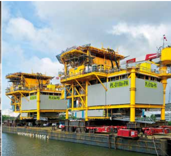
Two gas platforms delivered within one year
