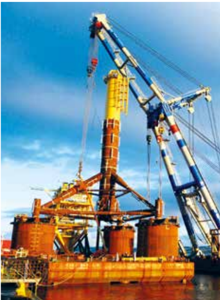
Re-usable platform with suction piles
