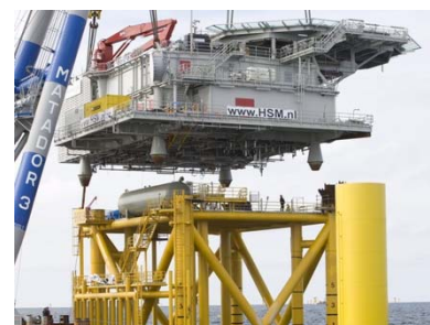
Horns Rev B - installation of topside
