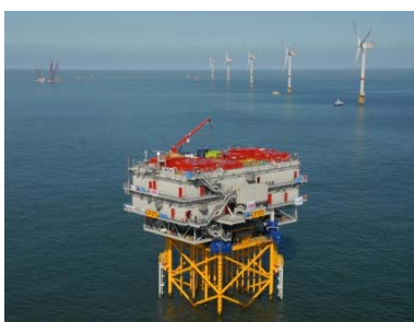
Thornton Bank - installed
