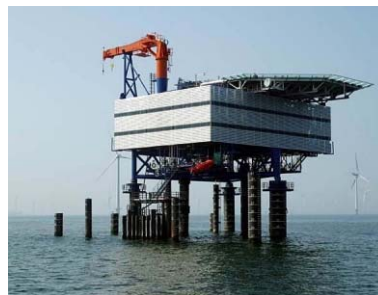
Horns Rev A - in operation
